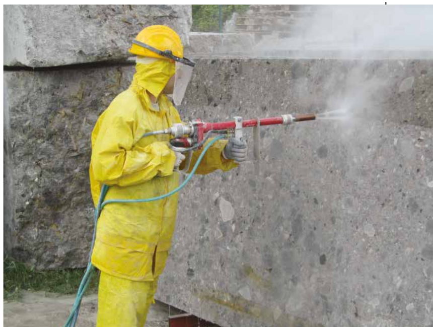
On-site treatment solutions using high-pressure manual application.
